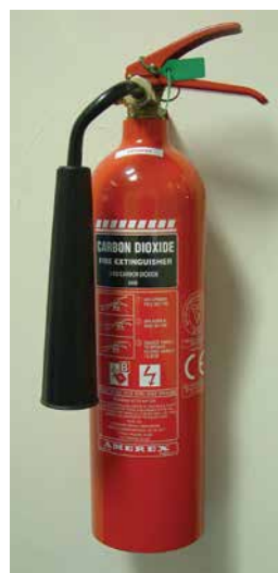
Figure 1.30 CO 2 Fire Extinguisher.
